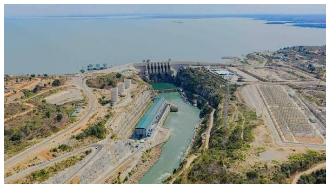
The Julius Nyerere Hydro-Power Plant in Tanzania.
